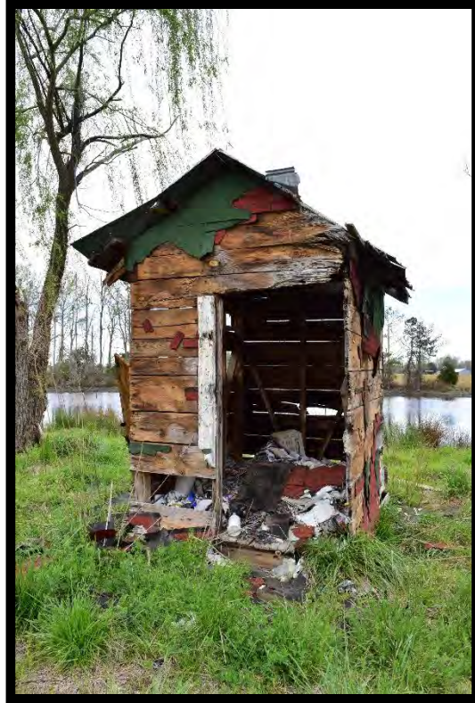
Figure 13: Barnes House, Shed.
