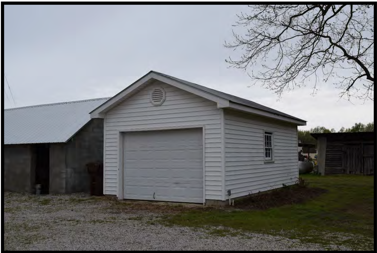
Figure 63: George Hinton House, Garage, Looking Northwest.
