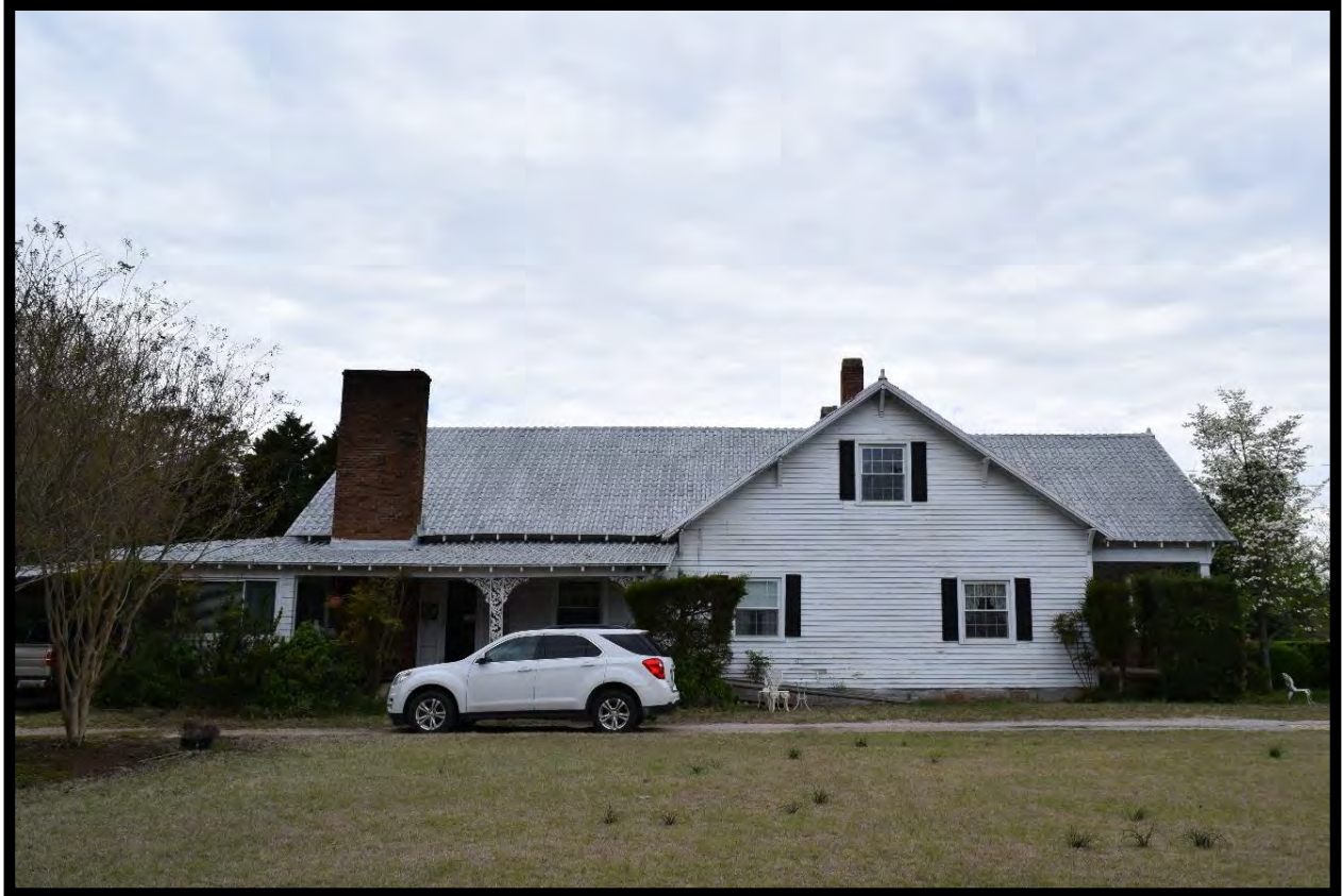
Figure 29: J. O. Barnes House, Looking North.
