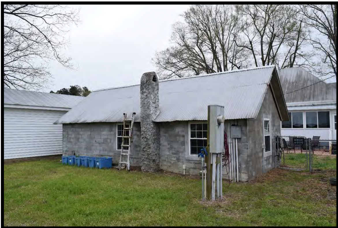
Figure 62: George Hinton House, Washhouse/Smokehouse, Looking Southeast.
