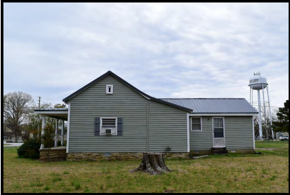
Figure 39: Wall House, Looking Southwest.
