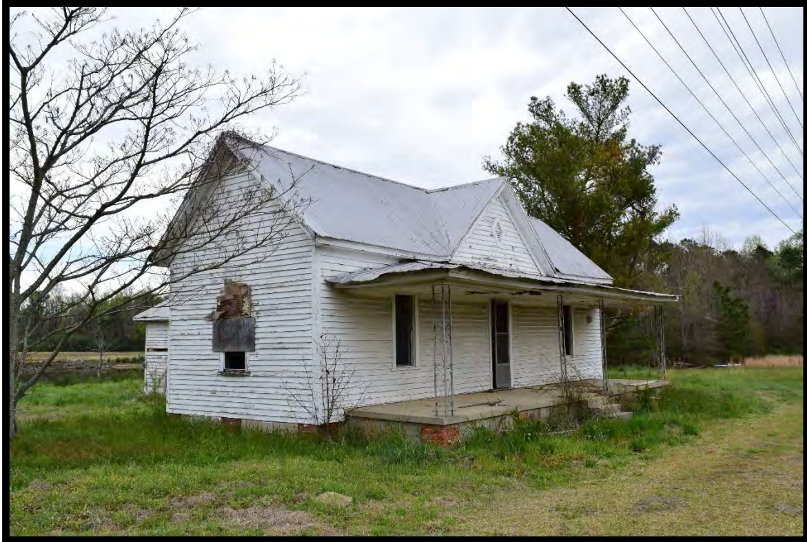
Figure 8: Barnes House, Looking Northeast.
