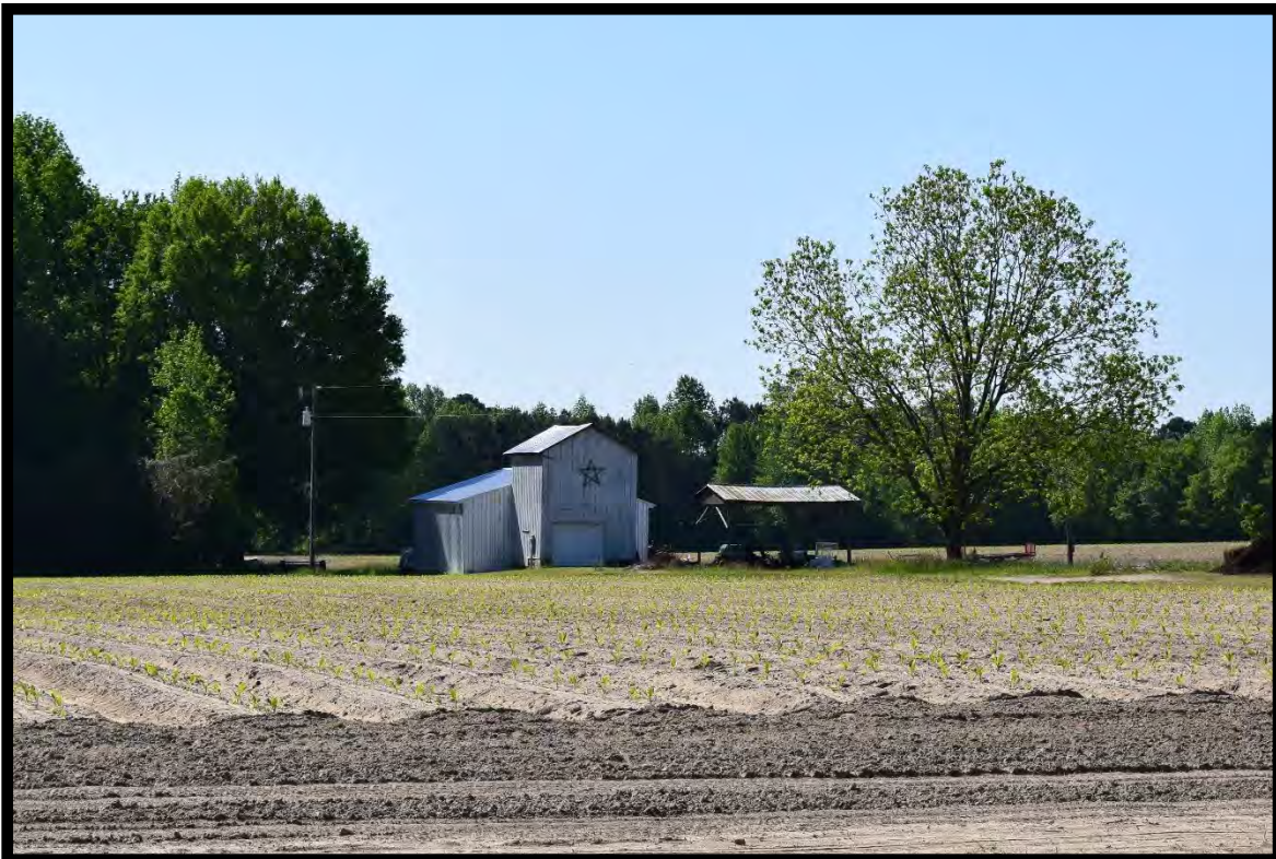
Figure 14: Barnes House, Tobacco Barn and Sheds.
