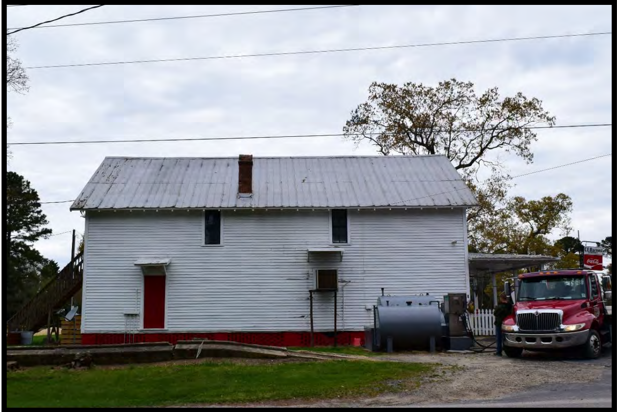
Figure 23: J. O. Barnes Store, Looking North.
