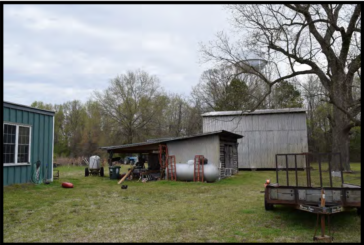
Figure 60: George Hinton House, Mule Stable, Looking East
