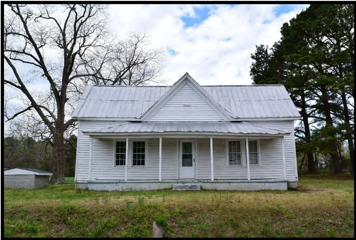
Figure 17: 2743 Castleberry Road, Archer Lodge, NC.
