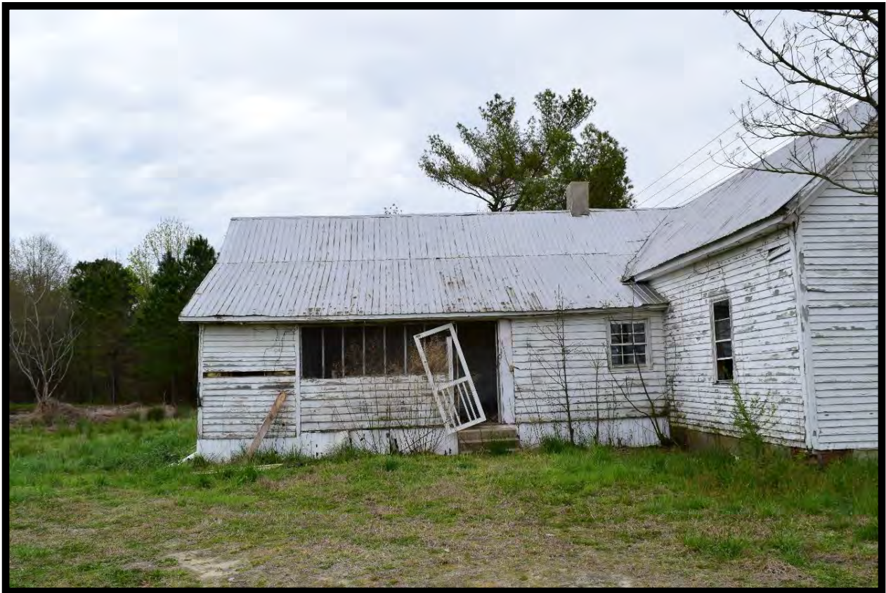
Figure 7: Barnes House, Looking East.
