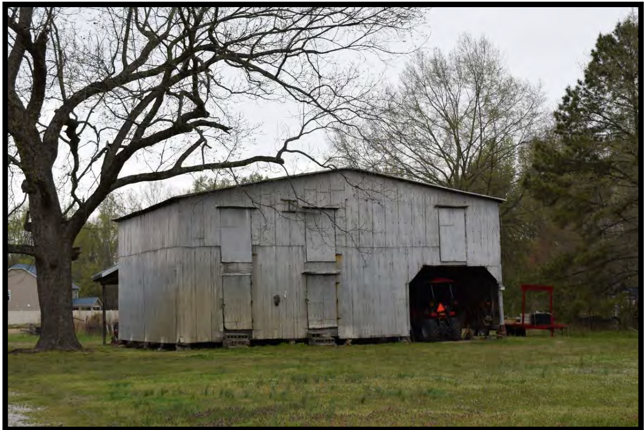
Figure 58: George Hinton House, Barn, Looking North.
