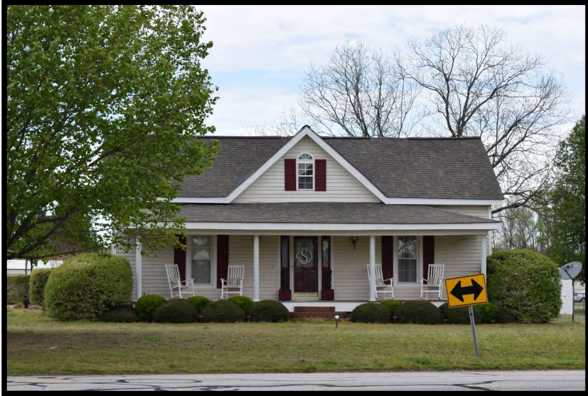
Figure 16: 6097 Covered Bridge Road, Archer Lodge, NC.
