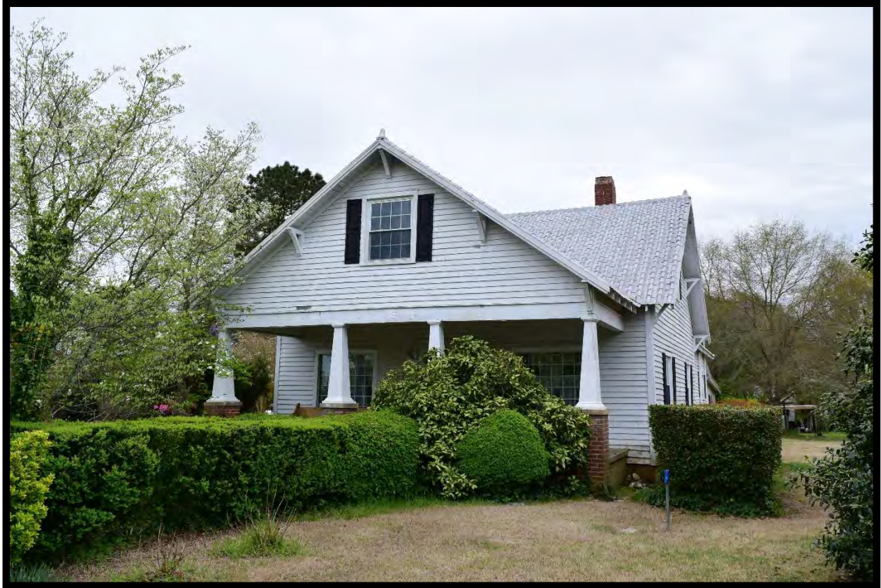
Figure 19: J. O. Barnes House, Looking West.
