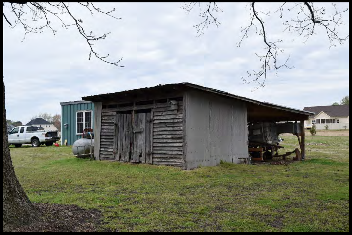
Figure 59: George Hinton House, Mule Stable, Looking Northwest.
